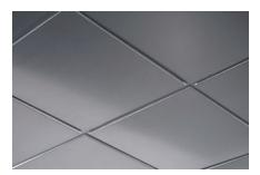
Drop ceilings are often used in renovation projects as efficient, economical ways to implement ceiling repairs that would otherwise be far more time consuming and labor intensive, and/or to reduce air conditioning and heating costs, and/or to conceal functional and structural components that may be undesirably visible along an existing ceiling surface.
